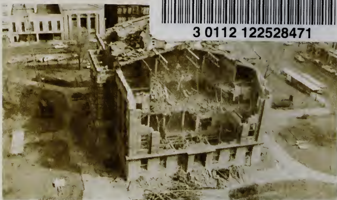
THE OLD BUILDING COMES DOWN, FEBRUARY 1966
